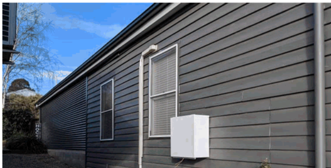
The use of timber and galvanised steel is a good and common combination in the village.
