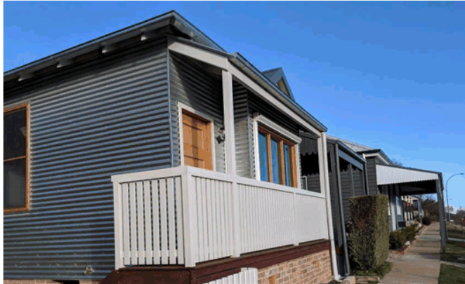
The use of timber doors and windows in the context of Galvanised steel cladding
