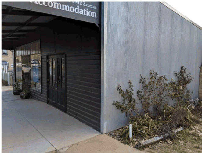
The use of vertical Mini-orb galvanised steel cladding has long been used in the Village on external walls.
